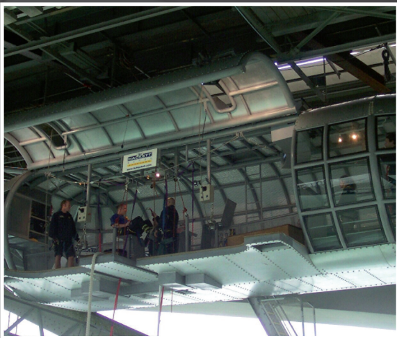
Auckland Harbour Bridge Bunge Pod - Space frame construction AJ Hackett
